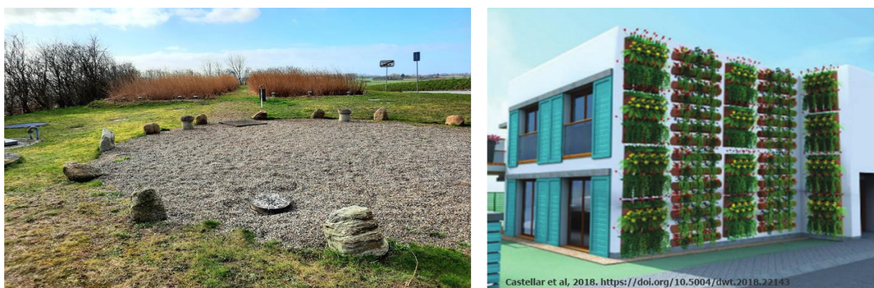
Figure 1. Treatment wetland in Denmark (project NATURE, left) and green-wall in Spain (project MULTISOURCE, right), designed to treat combined sewer of the area and greywater of the building, respectively
